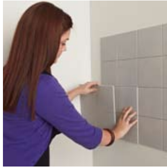
Take a second full panel and place it into the corner overlapping the tile
