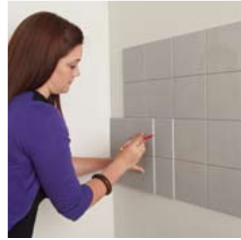
Draw a line where the two tiles meet. The piece you can see is the piece you need
