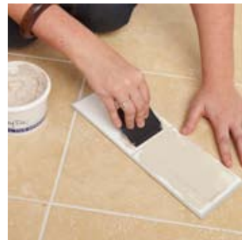
after test fitting, apply adhesive
