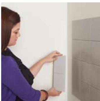
Offer into place with cut edge towards the corner
