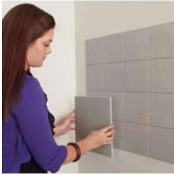
Place the tile to be cut over the last full panel.
